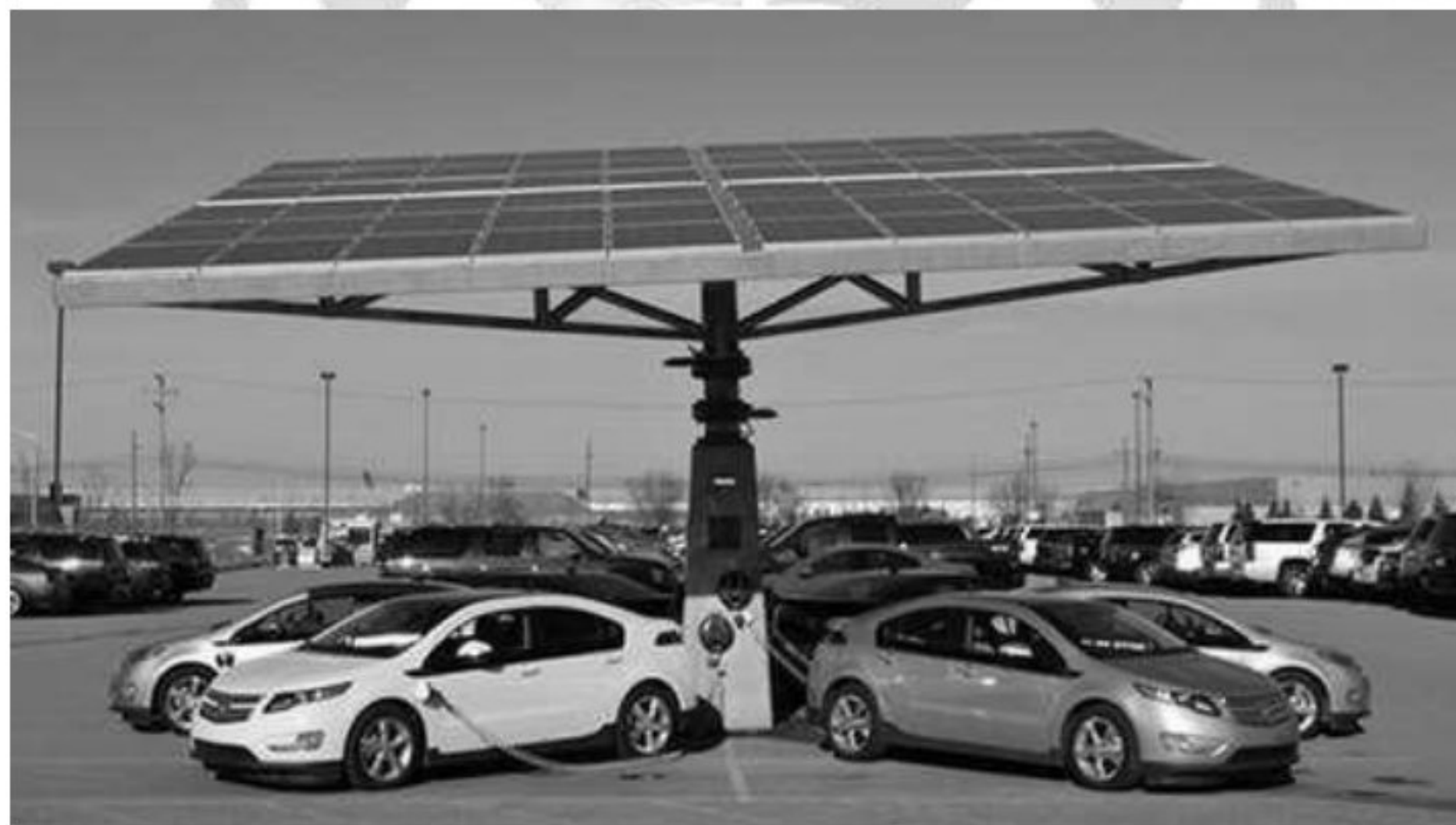
Fig 2: Self-sustaining solar EV charging station
